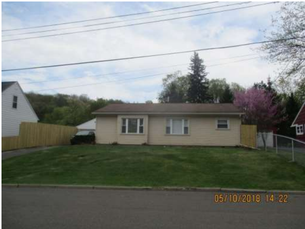
1 22 Lamont St as viewed from the north side of Lamont St.
