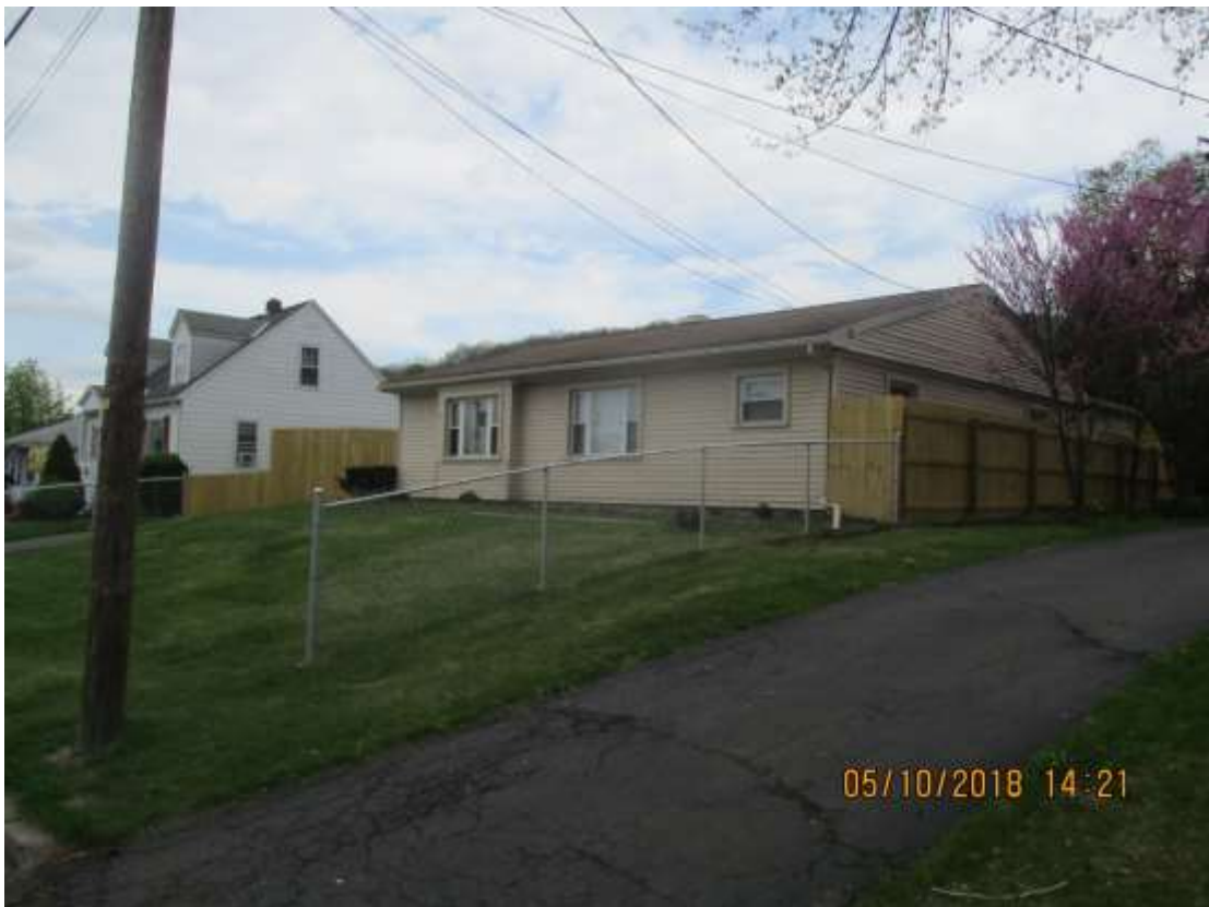
3 22 Lamont St and existing fencing. Viewed from the northwest
