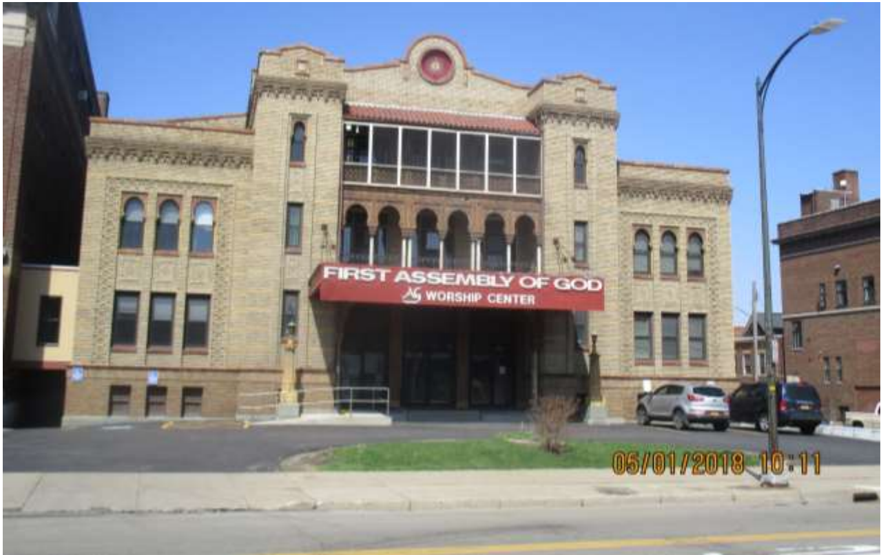
1 Facade of 255 Washington St. Location of proposed sign within the landscape island
