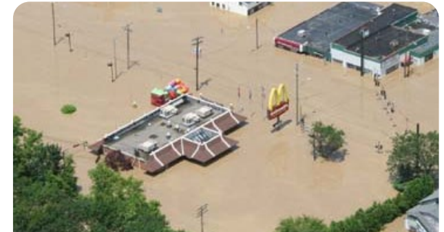
2006 Flood Court Street
