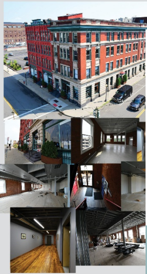
218-224 Water Street, Hull-Grummond Cigar Factory
