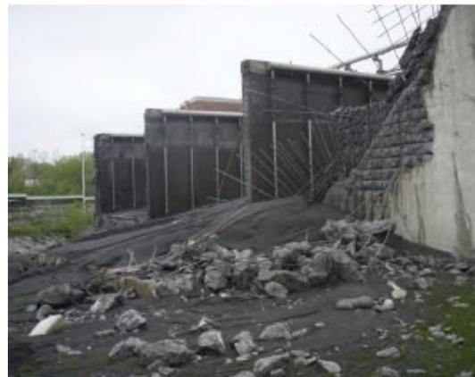
Collapse of bio-reactor unit wall at BJC WWTP (DEC photo)
