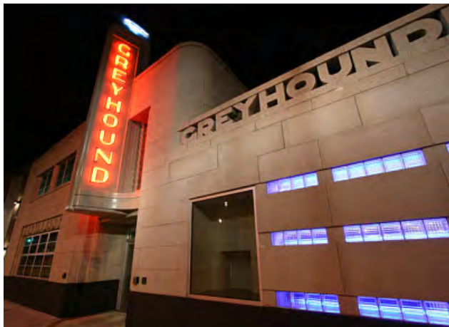
The Transit Center bus terminal serves as a gateway for regional and local bus passengers, and incorporates the historic Greyhound bus station building.
