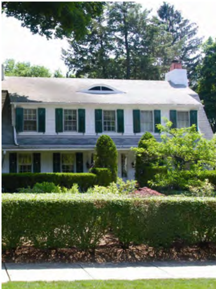
This Dutch Colonial Revival on Avon Road showcases a very large shed dormer, with a small eyebrow dormer above it.
