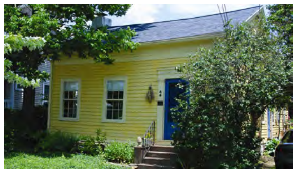
This Greek Revival structure on Oak Street retains high integrity with its original clapboard siding.
