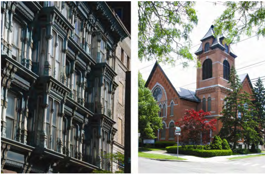
The Perry Building's highly ornate wrought iron façade and paint scheme and the Tabernacle Methodist Church's "bellcast" shaped tower roof and unique masonry work are character defining elements.
