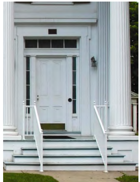
This Riverside Drive residence's front door is bordered by a transom and a pair of sidelights.
