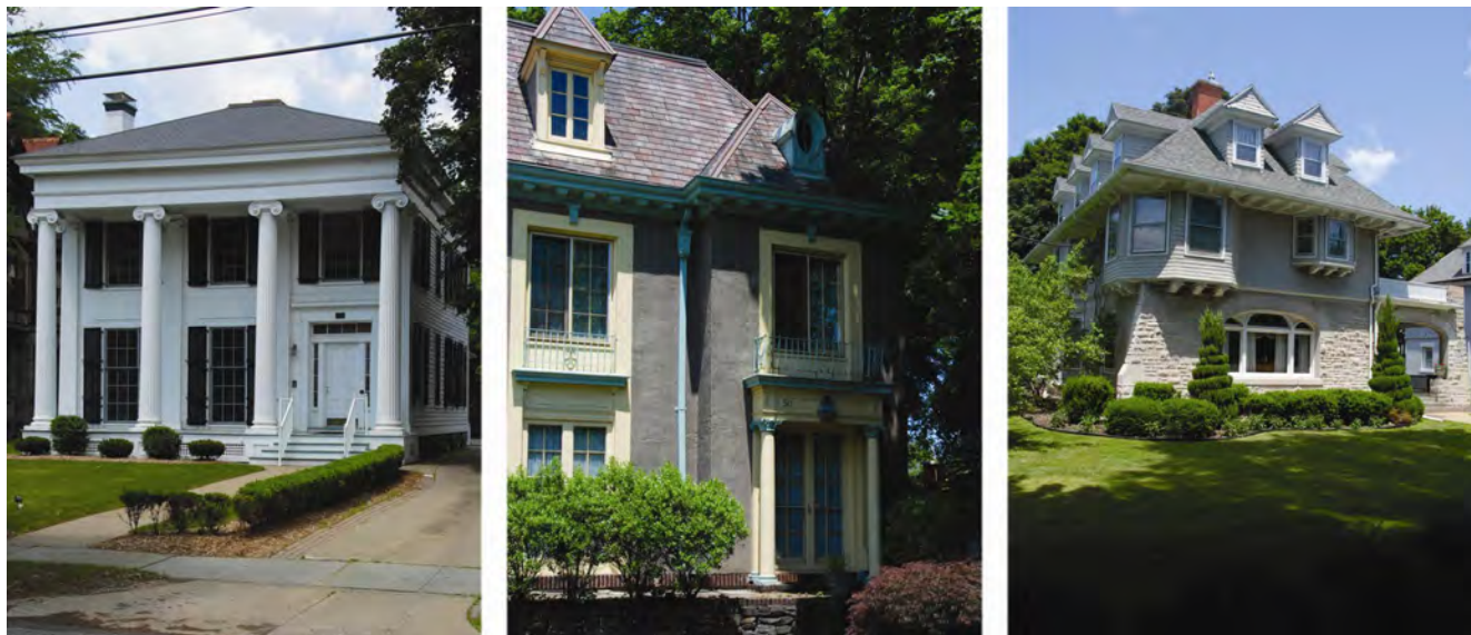
These three Riverside Drive residences utilize a hipped roof in a multiplicity of styles and applications.
