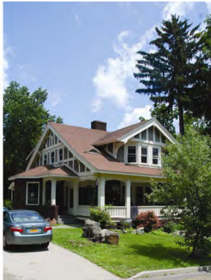
This Arts and Crafts Bungalow on Front Street has a large gabled dormer with complimenting eyebrow dormers to the sides.
