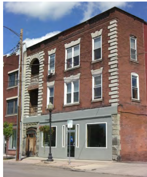
The character and integrity of this commercial structure has been compromised with an inappropriate first floor storefront modification, including use of incompatible materials, modifications to the building entry and a reduction in window transparency.
