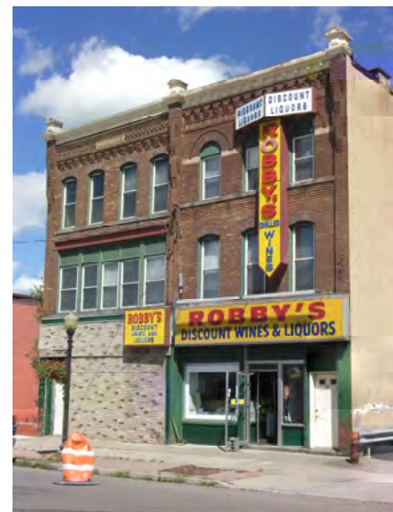
The building above represents both inappropriate storefront modifications and excessive signage.
