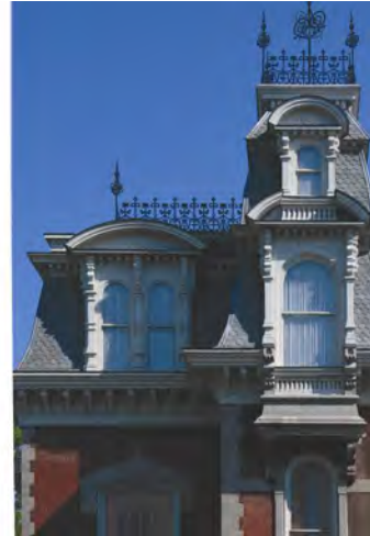
The rare cast iron roof cresting of the Phelps Mansion is a character defining element.
