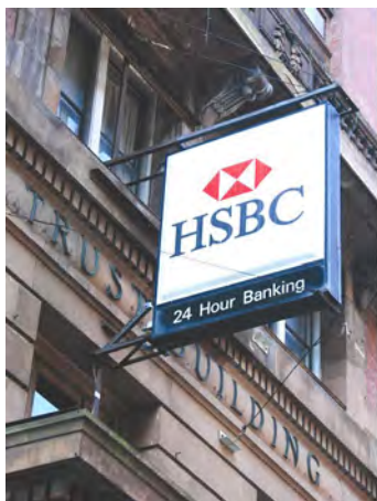
This sign's design clashes with its building's style and may cause damage to the stonework through its excessive network of bolts, plates and cables.
