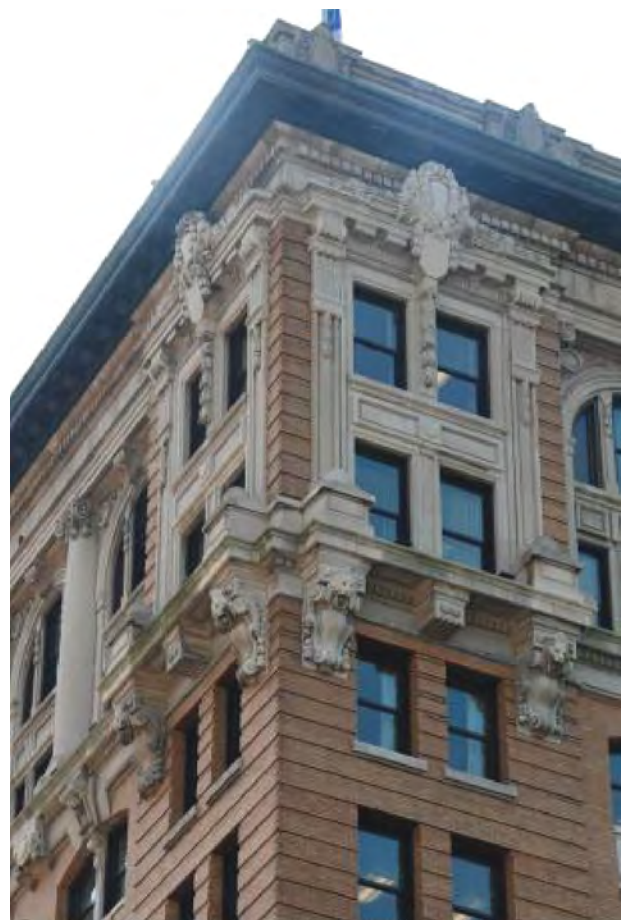
The Security Mutual Building is a local example of a masonry structure that has been well maintained.
