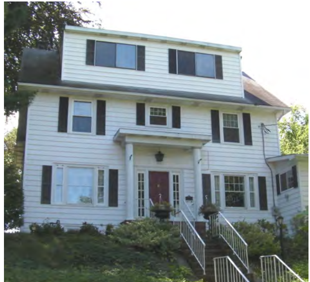
The character and façade of this traditional home have been altered by an inappropriate front rooftop addition. Its prominent placement, inconsistent windows and change in rhythm detract from the original design.
