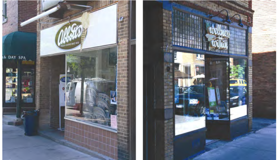
The building at left has been compromised through the inappropriate reconstruction of its storefront, signage that covers the upper transom and large fluorescent lighting.
