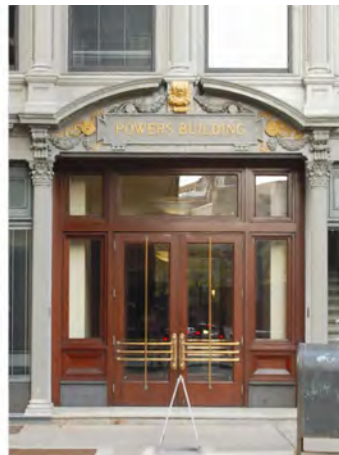
This reconstructed entryway to a Second Empire building complements the original façade with appropriate materials, arrangement, and details.
