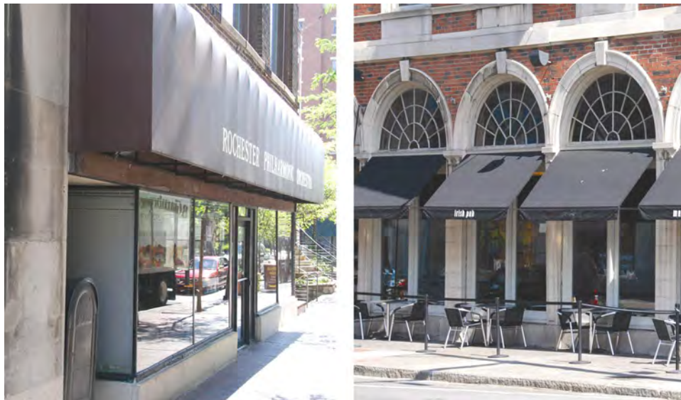
The character of the building at left has been diminished by the installation of an oversized, tall, fixed vinyl awning in addition to the reconstruction of its storefront.
