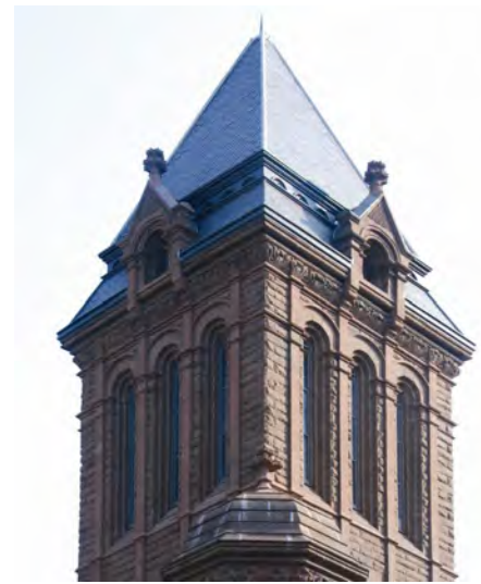
This distinctive Romanesque tower was restored with new copper ridging and matched slates, along with the relining of its built-in gutter.
