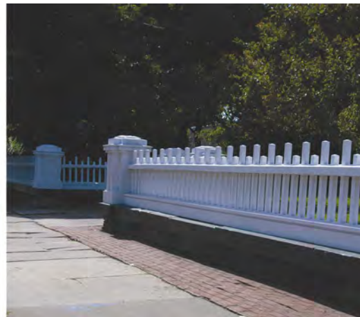
The fence above utilizes the original stone base in a historically accurate reconstruction of the original wooden fence.
