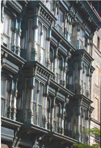
The Perry Building's cast iron façade is both decorative and structural.
