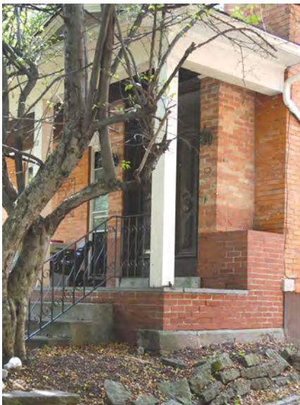
This residence's porch has been compromised through the removal of original brick and replacement with incompatible modern red brick.
