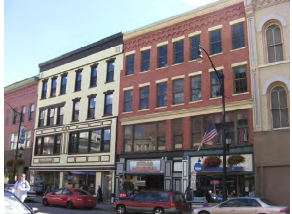
The series of commercial buildings above have retained their original arrangement of display windows, allowing for a high degree of transparency.
