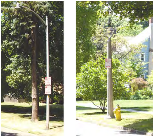
These views from the same residential neighborhood depict the importance of retaining historic lighting features. On the left the original street lights have been replaced by inappropriate vehicular oriented, aluminum, lights. On the right the original concrete, pedestrian scaled, harp lamps enhance the streetscape composition.
