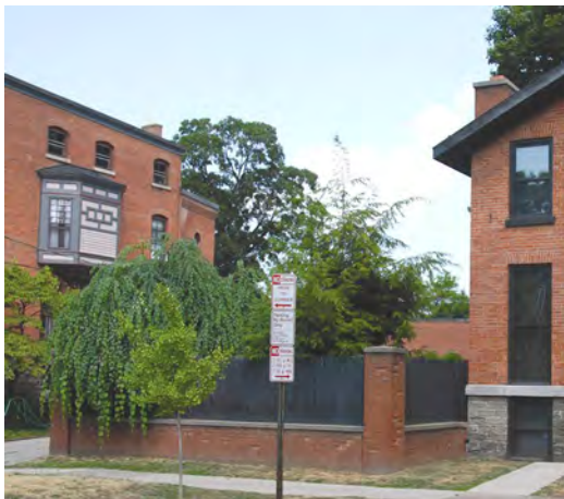
The fence above, while using brick, is inappropriate due to its height, lack of transparency, and relation to the adjacent historic home.
