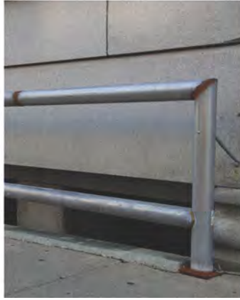
The original bronze railings of this building were replaced by inappropriate steel railings.
