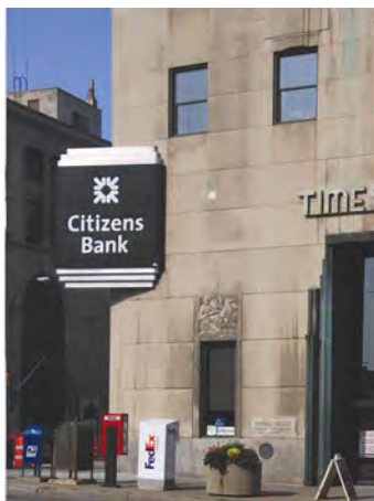
This sign, while complimentary in design to its Art Deco building, is inappropriate due to its size and building attachment.
