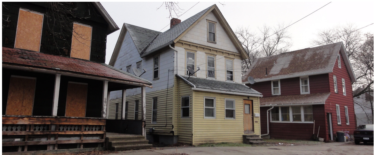
Homes in Need of Repair
