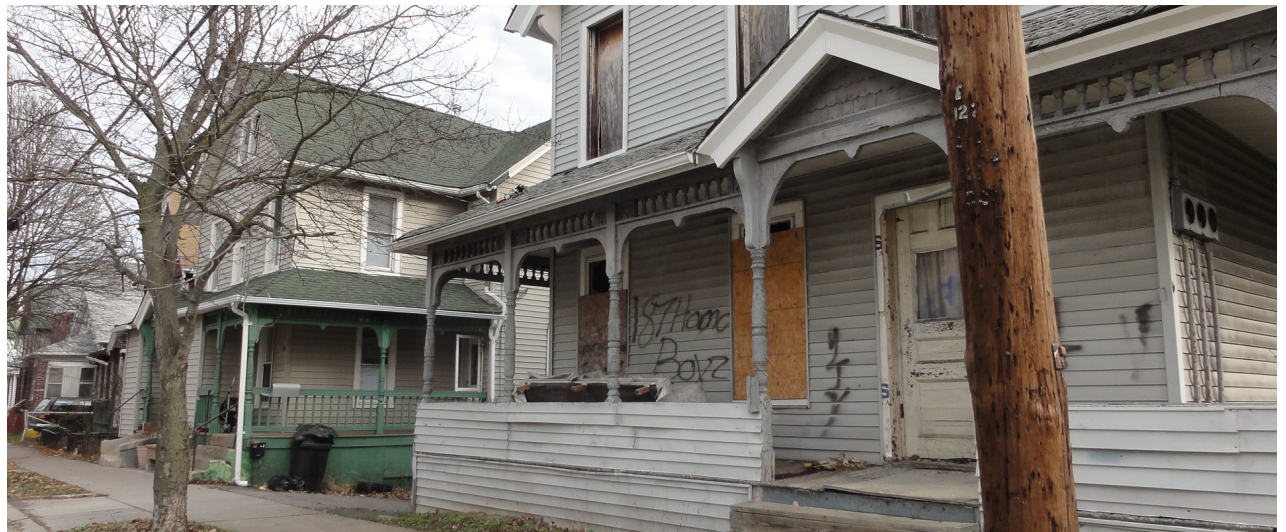
Vacant Home in the North Side
