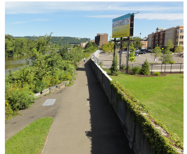
Chenango Flood Wall along the Riverwalk
