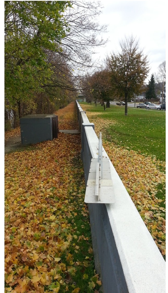
Susquehanna Flood Wall along North Shore Drive
