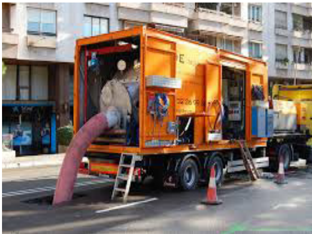
Trenchless road reconstruction
