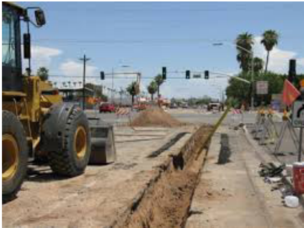
Trenched road reconstruction
