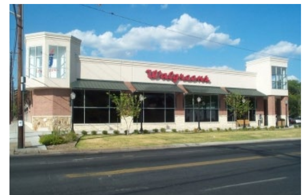
MORE PREDICTABLE AND PRESCRIPTIVE ZONING STANDARDS ARE NEEDED FOR THE CORRIDOR. UNDER C-1, EITHER ONE OF THE ABOVE WALGREENS IS ACHIEVABLE, BUT FROM A WALKABILITY PERSPECTIVE THEY ARE VERY DIFFERENT.
