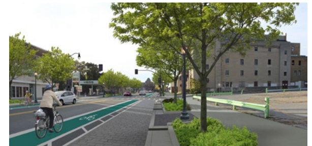
OPTION 2. TO HELP CAPTURE AND CLEAN STORMWATER, ON-STREET PARKING INCLUDES PERVIOUS PAVING AND TREE WELLS INCORPORATE VEGETATED BIO-SWALES.
