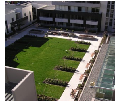
AN EXAMPLE OF AN INTERNAL COURTYARD.
