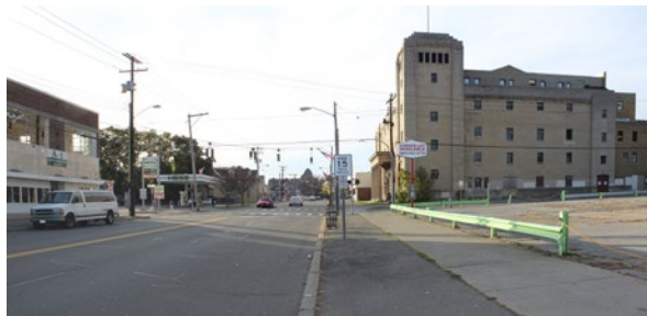
EXISTING CONDITIONS. MAIN AND MURRAY LOOKING WEST.
