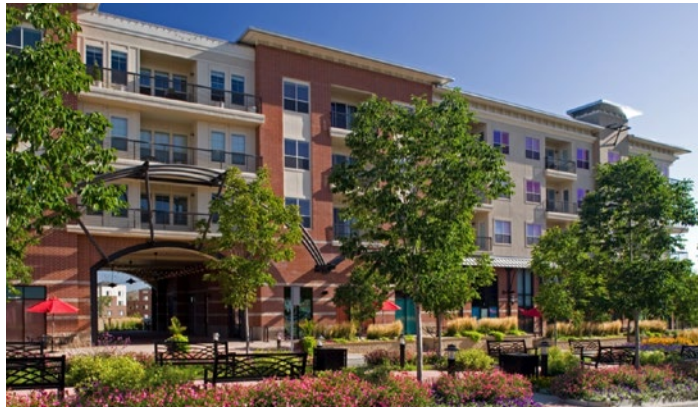
AN EXAMPLE OF A 4-STORY MIXED USE BUILDING THAT COULD FRONT MAIN, REPLACING THE SURFACE PARKING LOT THAT EXISTS TODAY.
