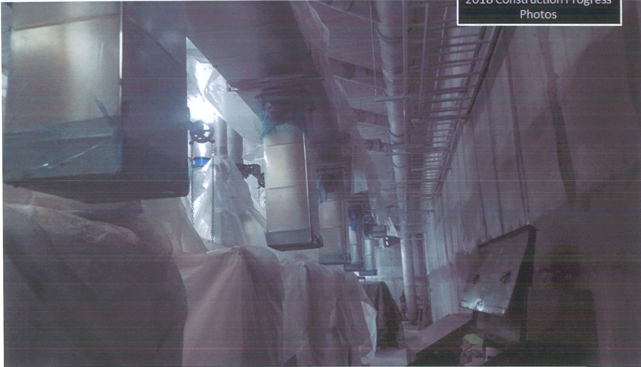
Blower Building – Duct Work Installation on Blower Units
