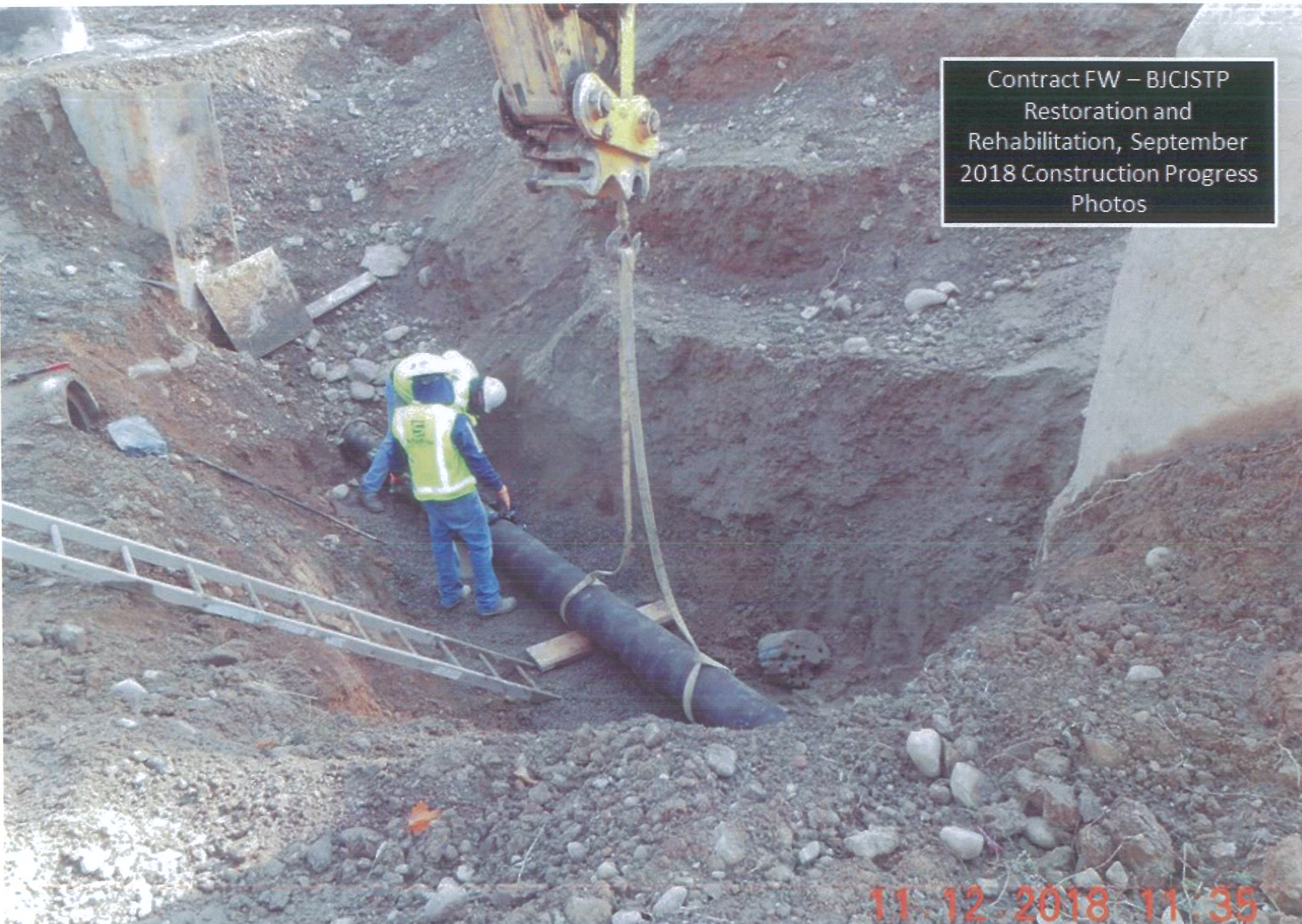
Manhole 1 Redirection to Manhole 2
