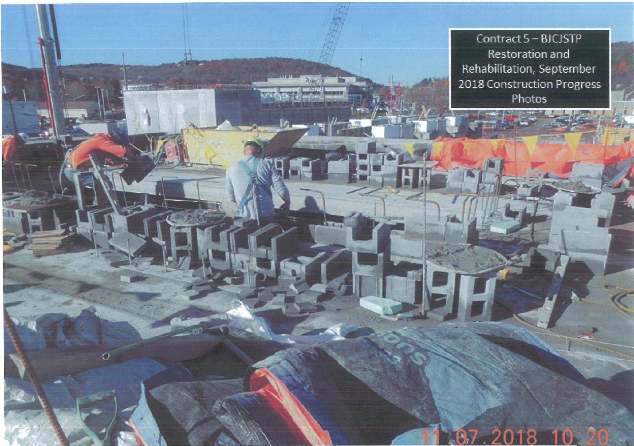
Headworks Facility – Skylight Walls Masonry Block Installation
