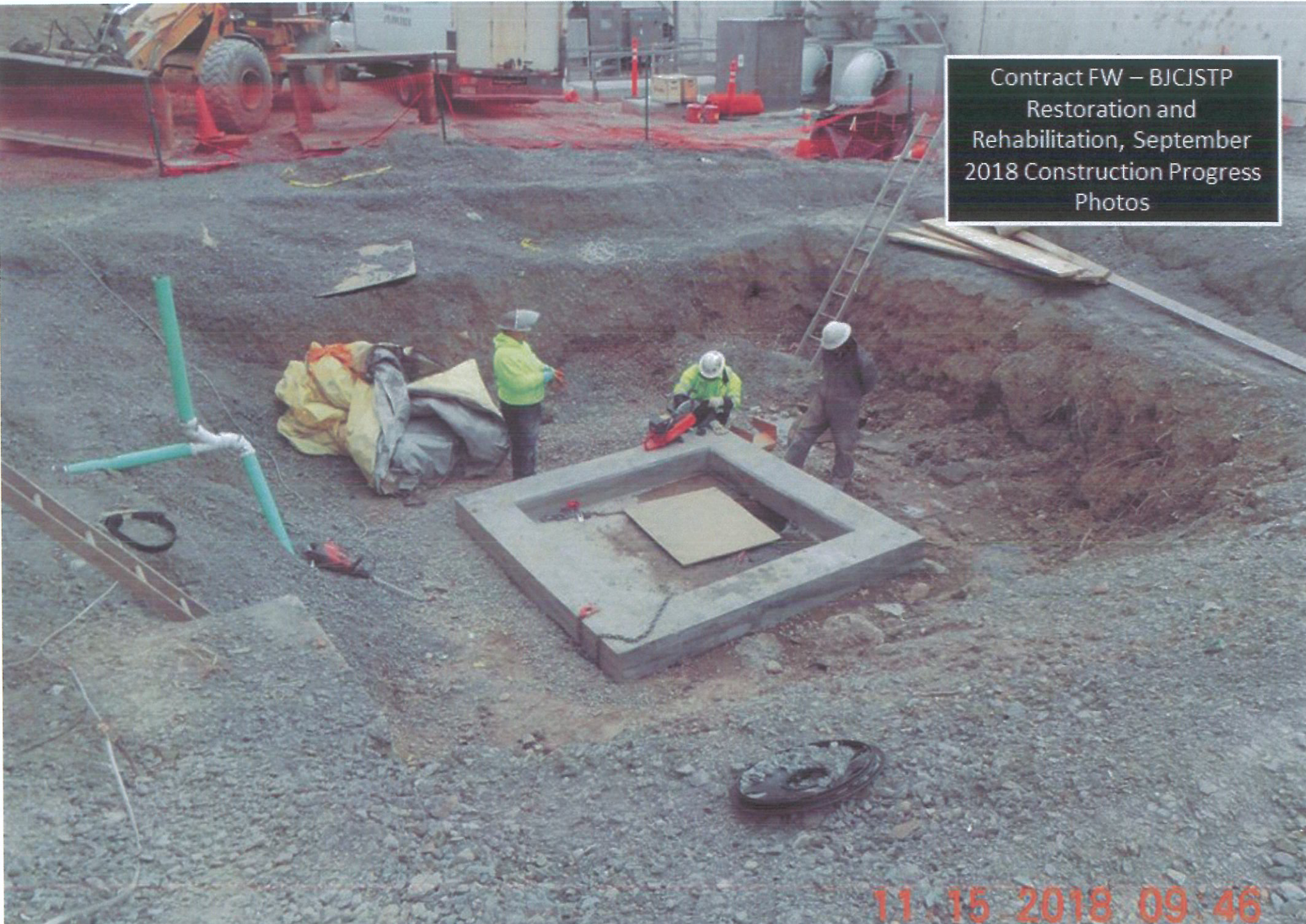
Sampling Manhole Cover Being Cut to Access Below
