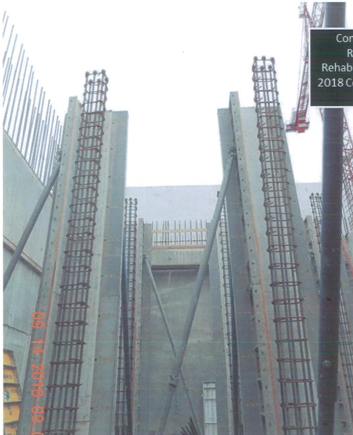
CN 9-14 – Cell 13 Column Reinforcing Steel and Partial Form Work
