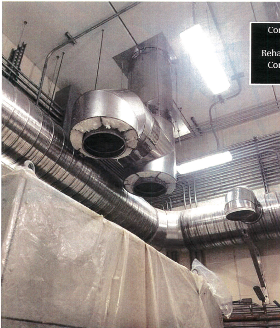
Sludge Processing Building – Installation of Micro Turbine Breeching
