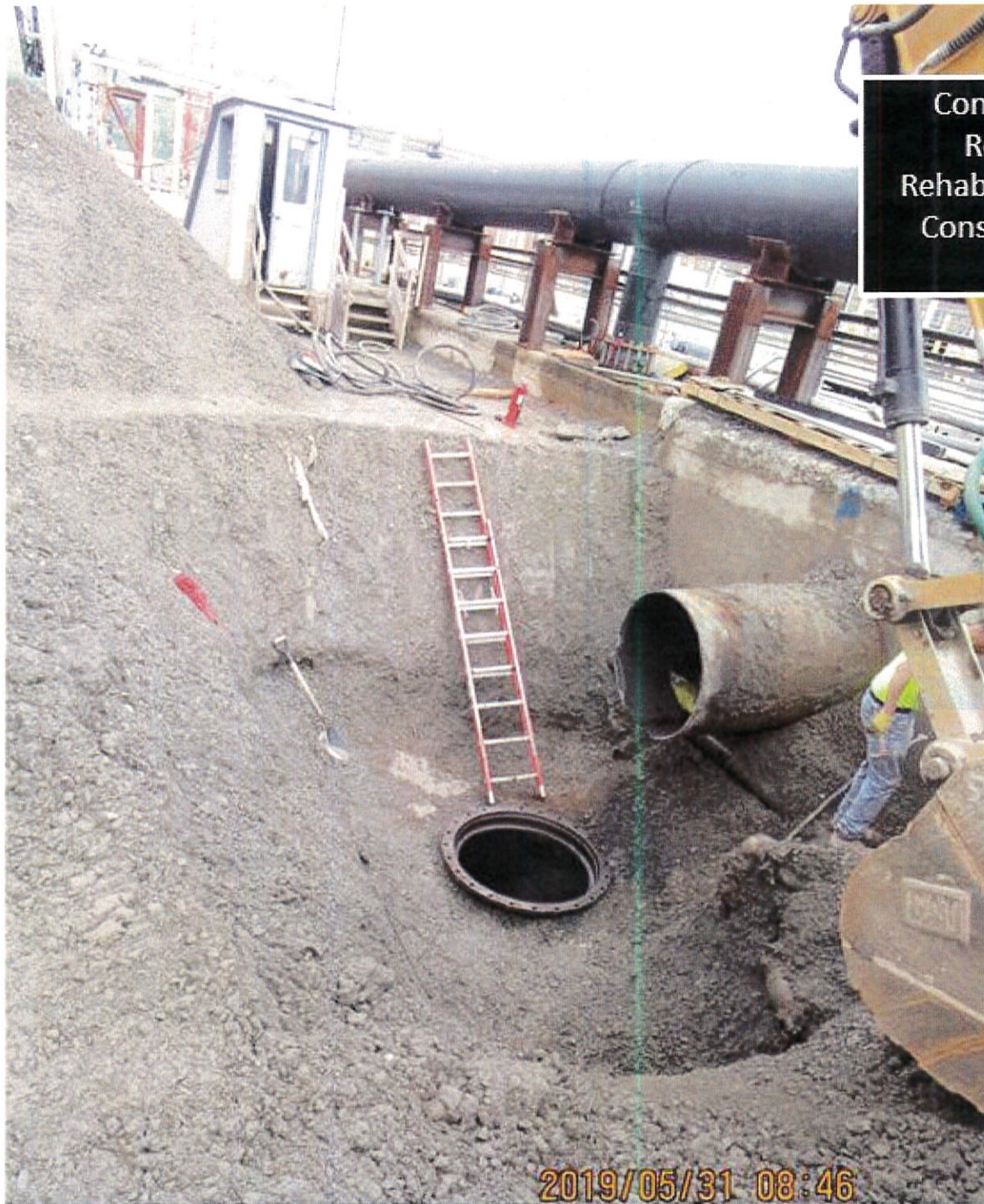
Primary Distribution Box 1 – 36 Inch Line Installation Progress Photo
