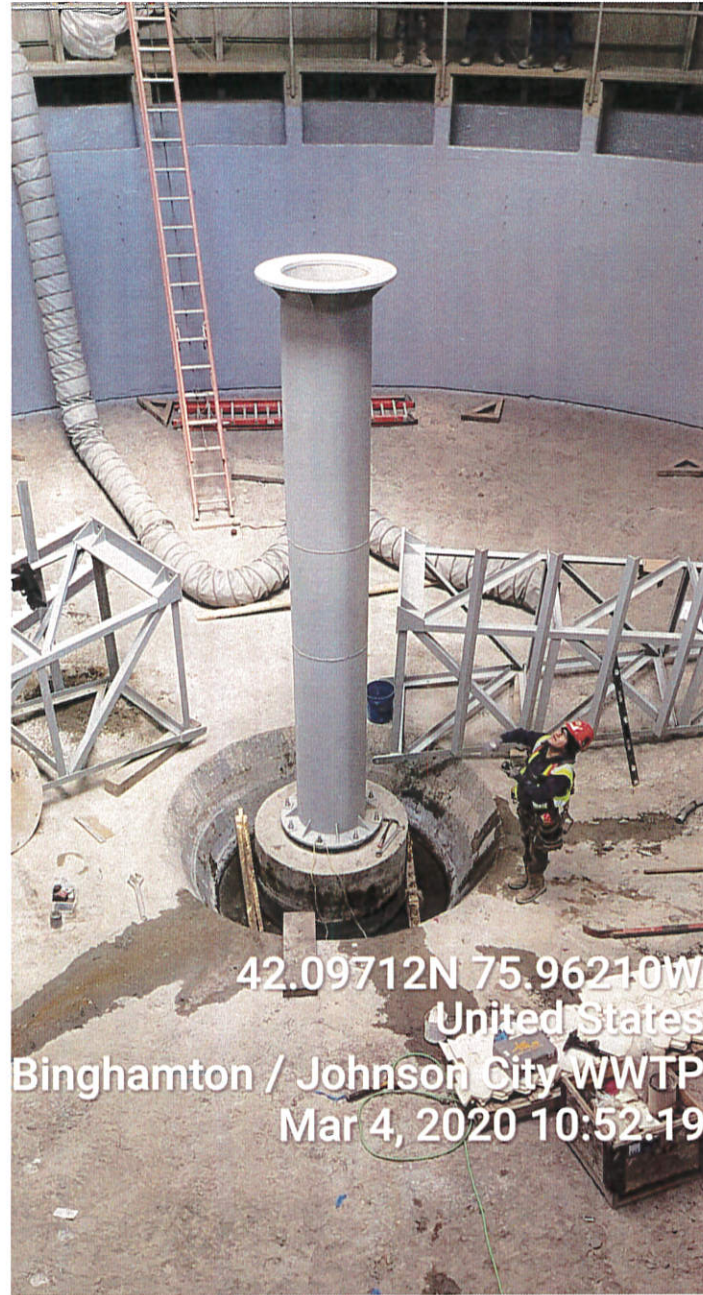
Installation of Pedestal for Thickener #2
