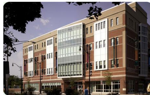
Binghamton University's Downtown Center at 67 Washington St, Binghamton earned LEED Silver Certification
