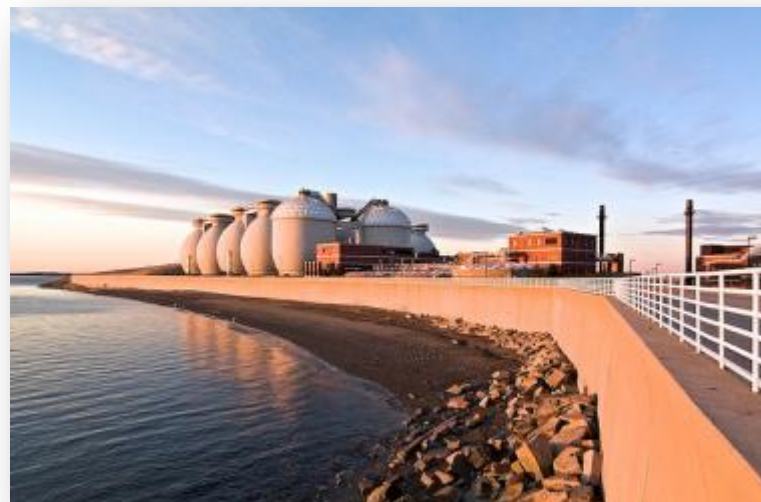
Sludge digesters process sewage sludge to extract methane for energy generation at the Massachusetts Deer Island Waste Water Treatment Facility.
