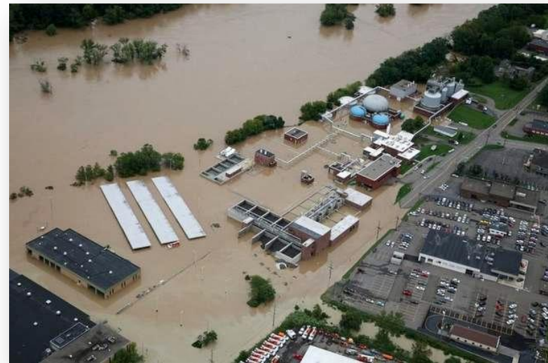
Binghamton-Johnson City Joint Sewage Treatment Plant in Vestal during the 2011 Flood
