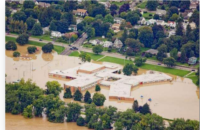
Binghamton's MacArthur Elementary School during the 2011 Flood
