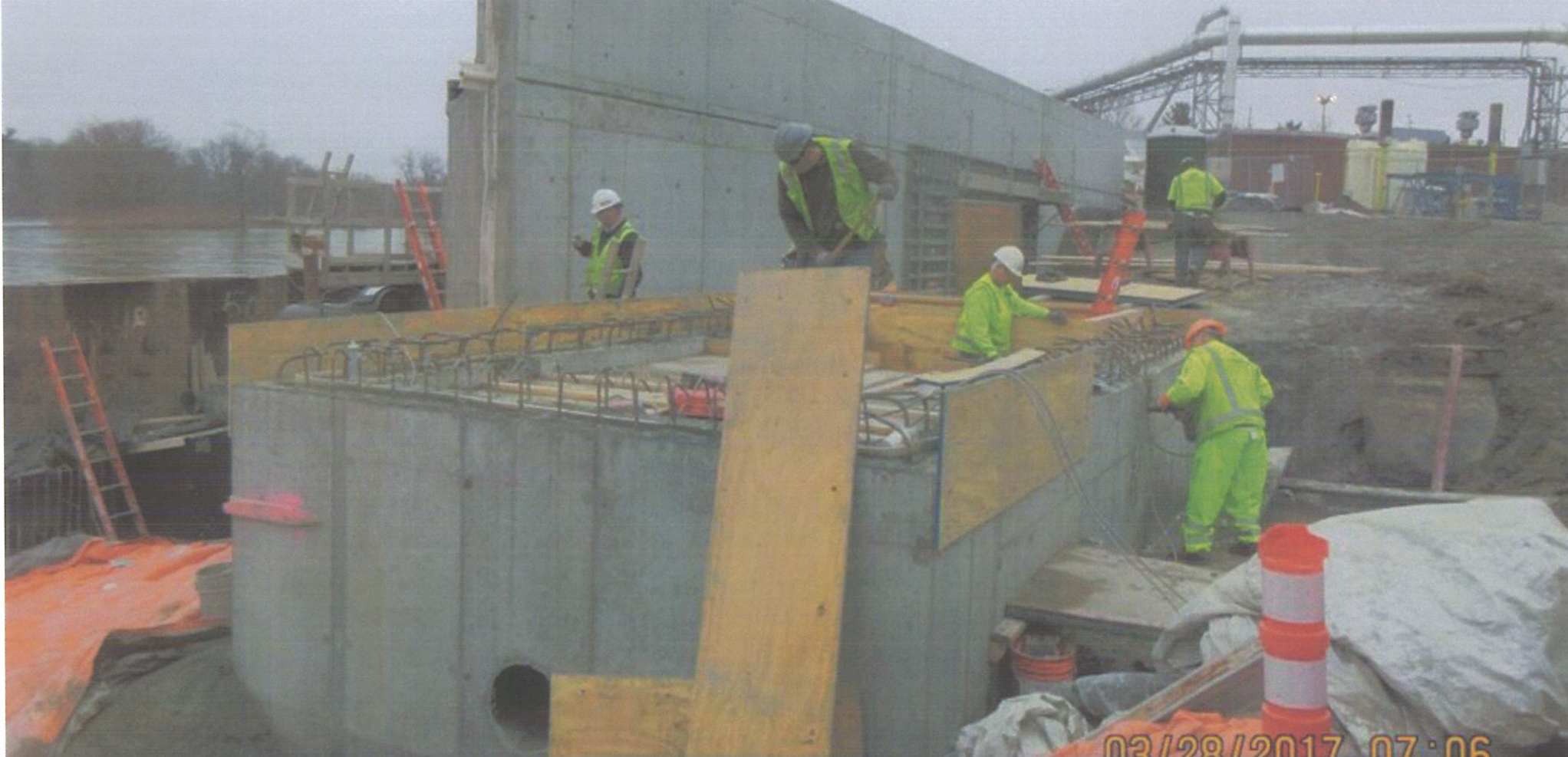
Forming of Suspended Slab for Pumping Station No. 2 (West End)
