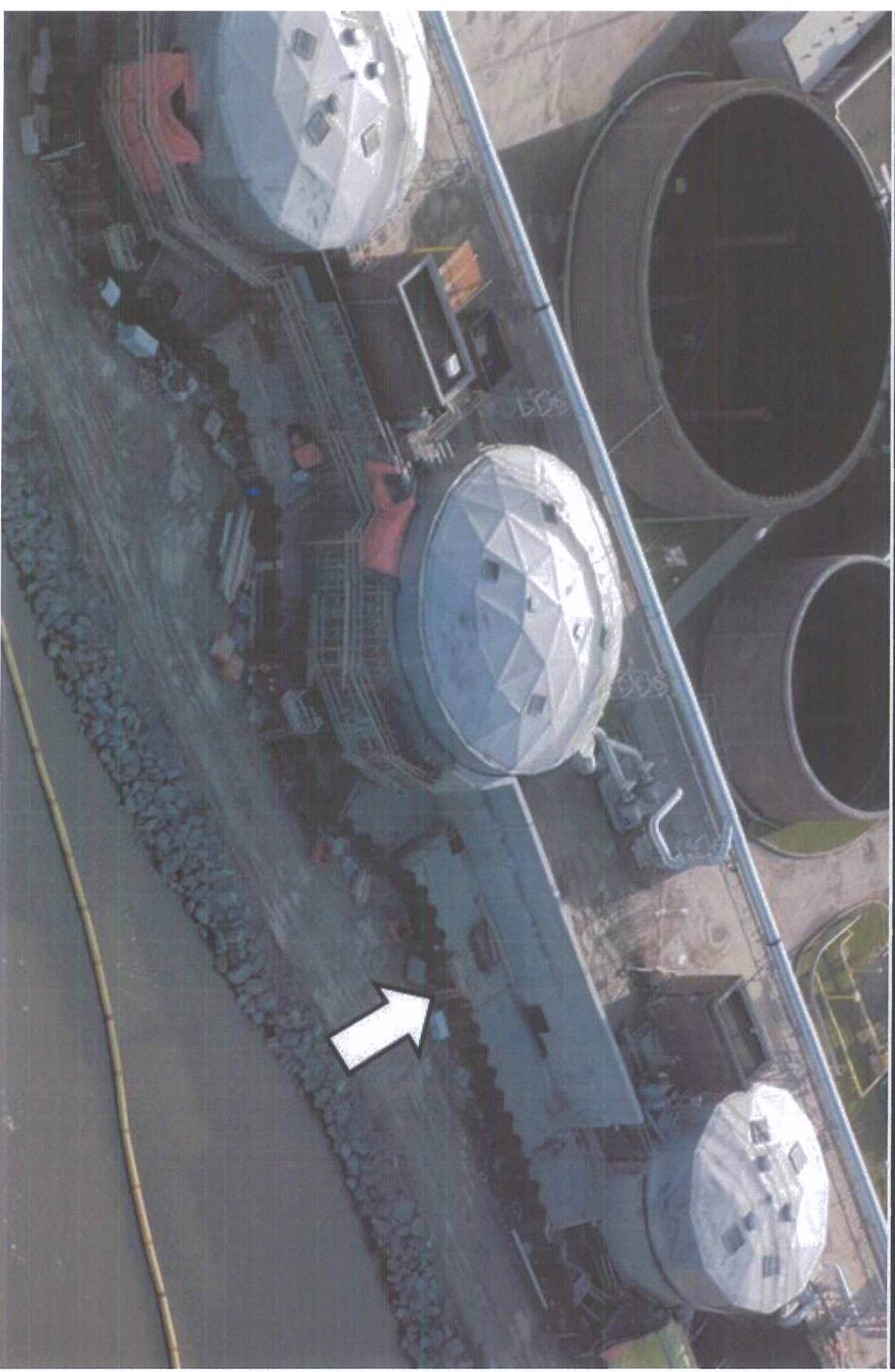
Aerial View of Completed Sections of the Floodwall, Indicated by Arrow
