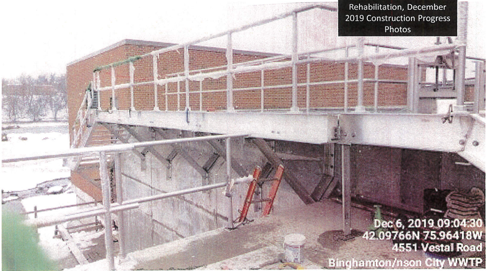
DN to UV Building Walkway Installation
