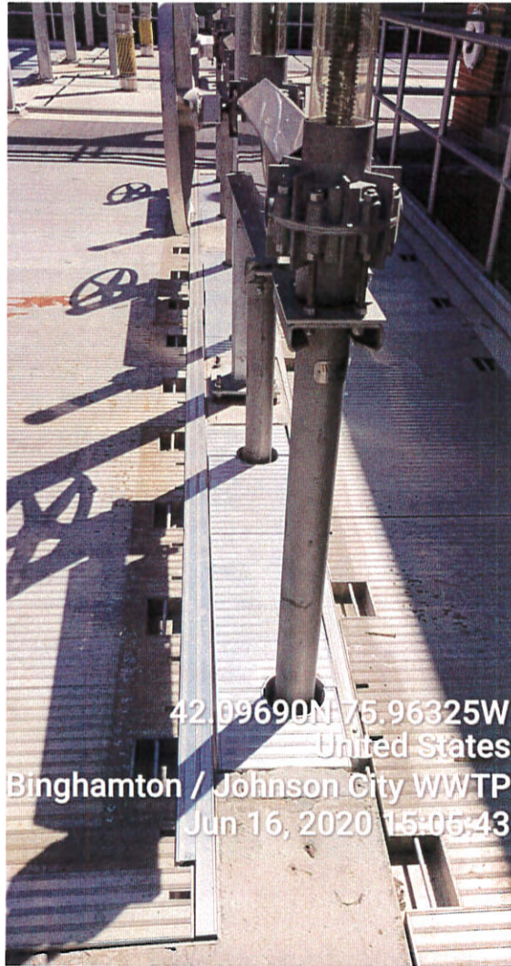
Headworks Distribution Box new Grating for Slide Gates
