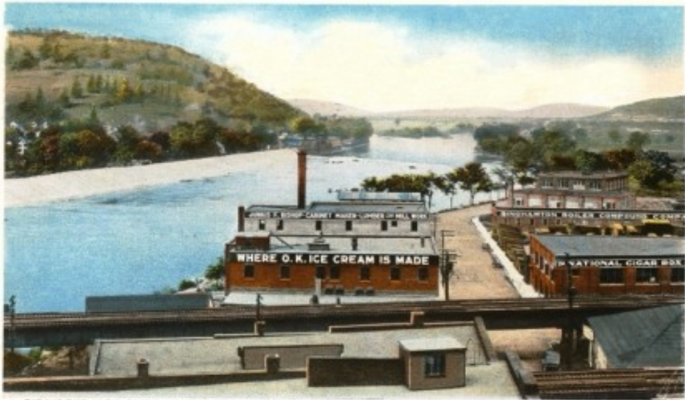
BIRD'S EYE VIEW CHENANGO RIVER AND DIKE, BINGHAMTON, N. Y.
